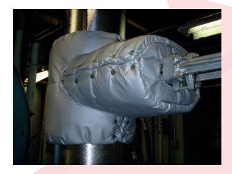
INSJACK-F® jet fire resistant jackets have been tested in an extensive range. It means INSJACK-F® may be used on a wide variety of fittings and equipment such as; piping, flanges, valves and actuators, vessels, heat exchangers, pipe supports and control panels.
